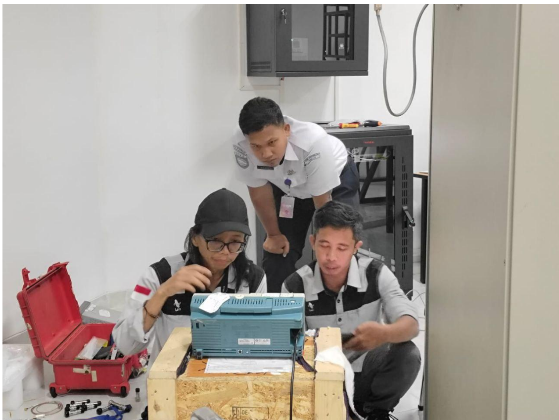
Gambar 35 Kegiatan Corrective Maintenance Radar Cuaca Sintang
